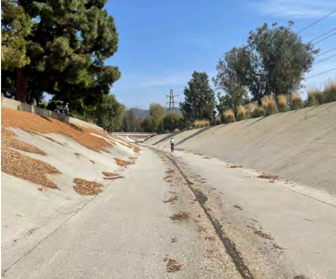
Changes to the cross section could be considered for trapezoidal sections of the channel
