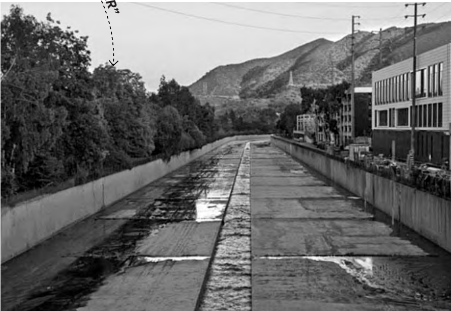
typical condition, post-channelization one of the standard segments of the Verdugo Wash, which was created to mitigate and divert waters from large-scale flood events
